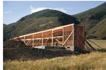
1. View of a study model, ca. 1968 2. Interior view of the staircase 3. General exterior view 4. South elevation, May 1971 5. Construction site view of the balloon-frame skeleton, ca. 1969 6. Axonometric views of the project phases between 1968-72
